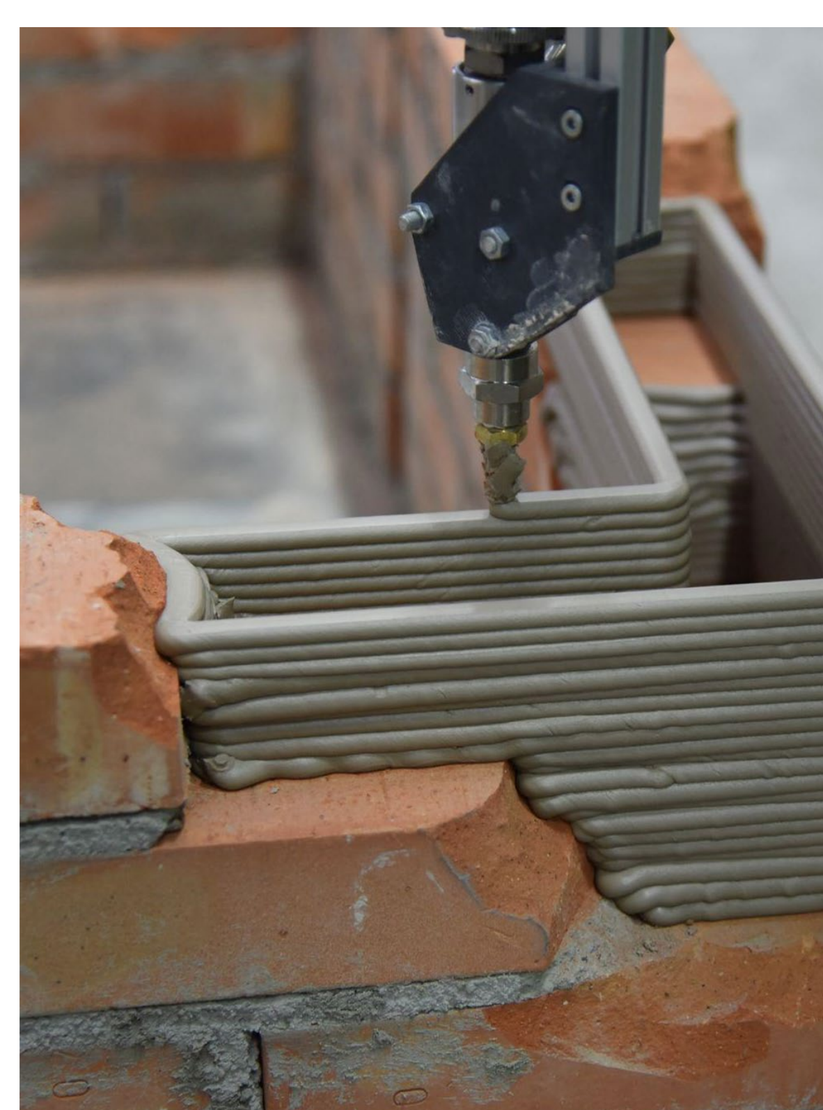
Figure 14: In situ repair of existing building components, shown using clay extrusion.
