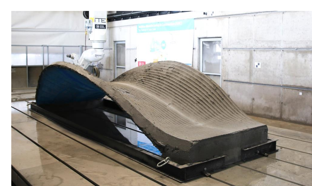
Fig 10: Knitcrete bridge demonstrator
